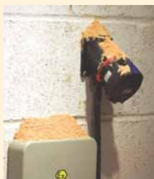
Plugs and socket-outlets intended for use in the presence of flammable dust, either in suspension or accumulated, must be protected against dust ingress.
