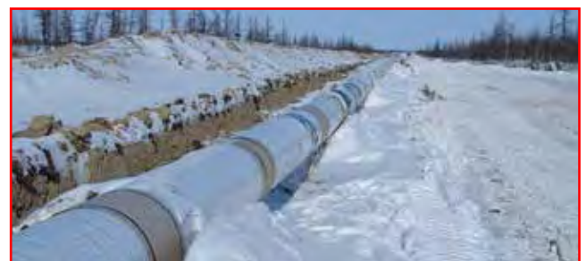
Completed Skin Trace system prior to burying
