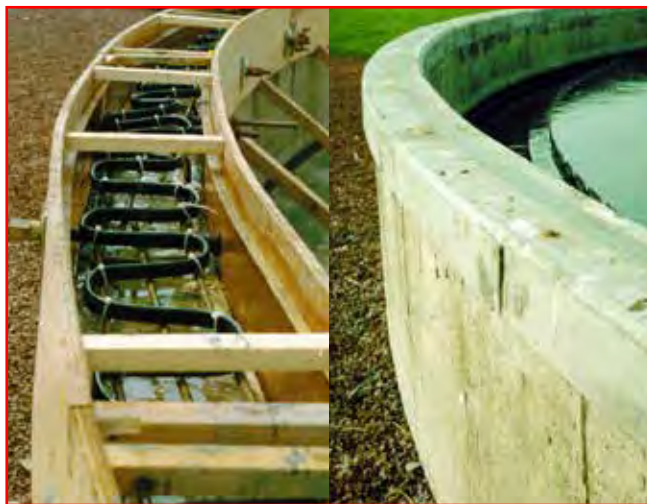
Final Settlement Tank de-icing
