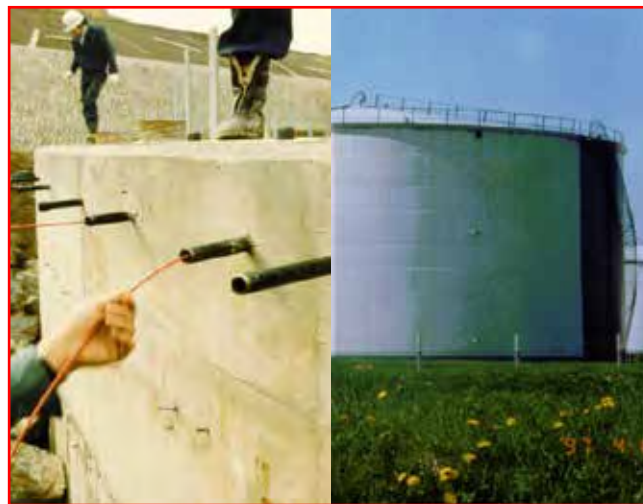
Tank base heating
