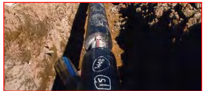
Buried, Pre-insulated Pipe with Longline HTS3F
